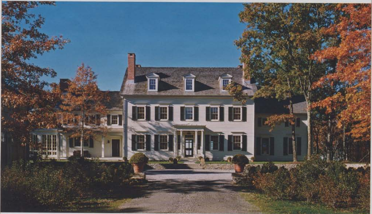
A new 8,500-sq.-ft. house and outbuildings by New York City-based G. P. Schafer Architect, PLLC, draw on local Hudson Valley precedents — and utilize materials from an existing Federal farmhouse — to create an authentic, sustainable family home. All photos: Carter Berg
