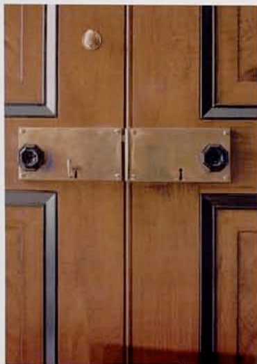
E. R. Butler created custom hardware for the residence, including these cobalt blue crystal doorknobs that were used throughout the apartment. They are from one of Butler's 19th-century reproduction lines. The entry doors were fitted with double brass rim-locks and a large nickel silver key thumb turn.
